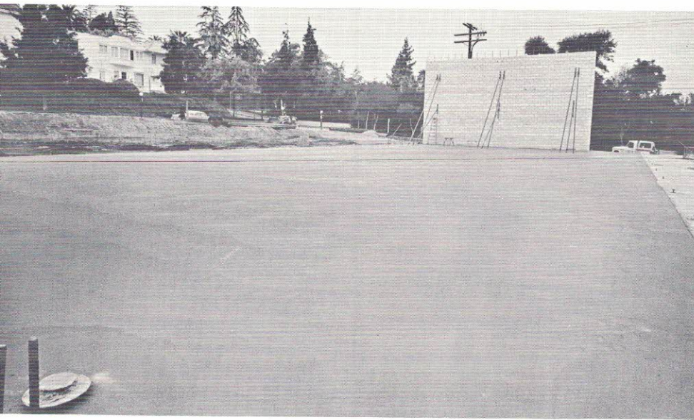
Foundation floor for gymnasium already poured.
